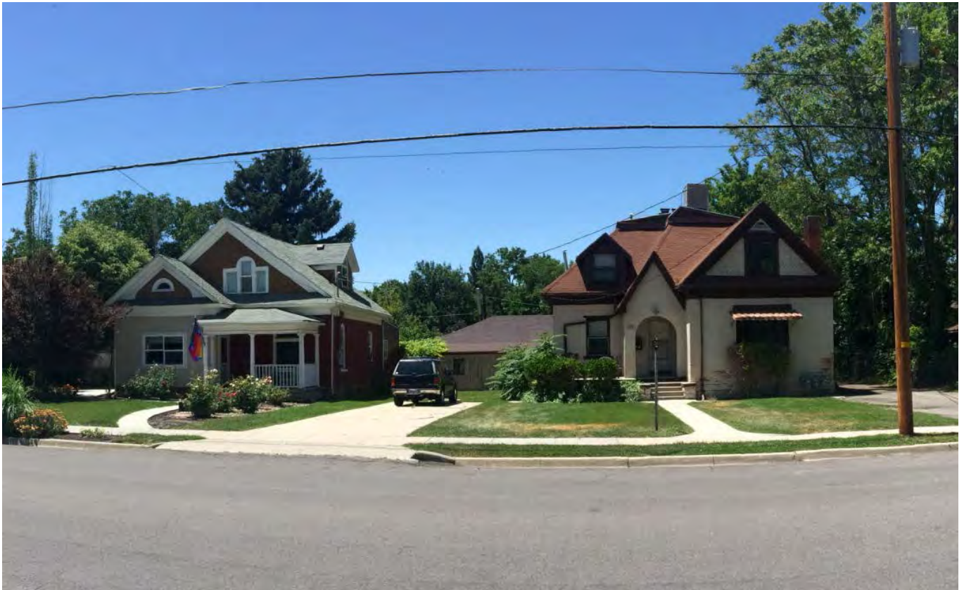
Existing development to the north of the subject properties
